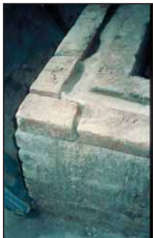
Figure 25 Corner of a Bricks and Sand Cool Chamber
