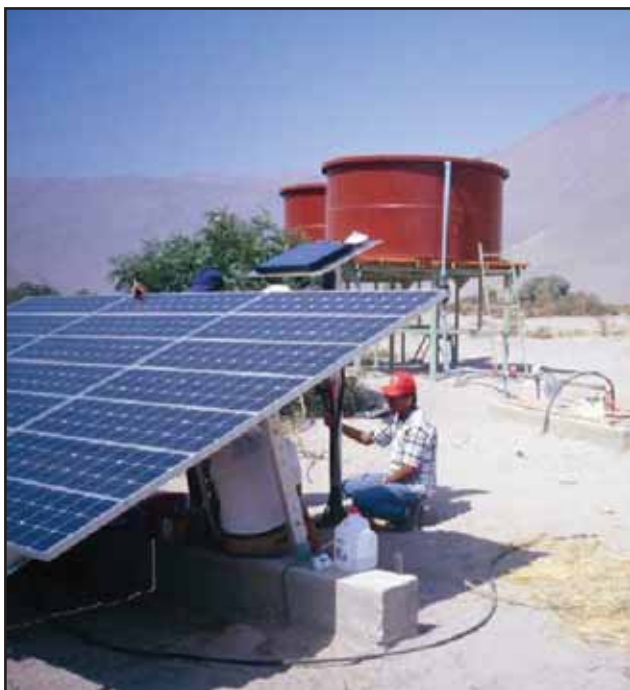
Figure 2 Solar-powered Drip Irrigation System in Chile
