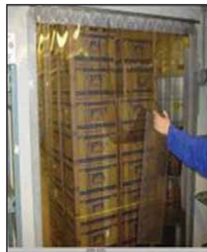
Figure 29 Plastic Curtains to Keep Cold Rooms Cold
